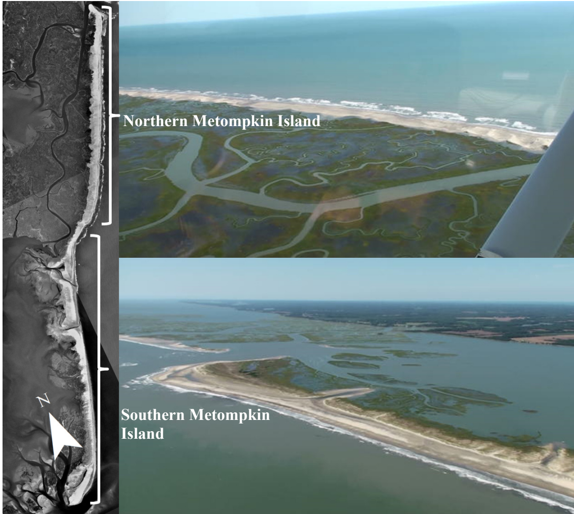
Figure 1.5: Orthorectified image of Metompkin Island in 2002. Inset oblique aerial images collected following Hurricane Irene in 2011 (photo credit: John Porter, 2011).
